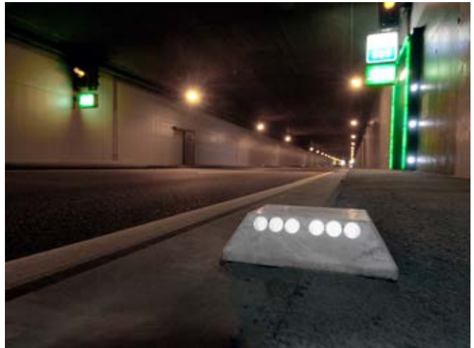
Tunnel St. Maurice, Wallis
