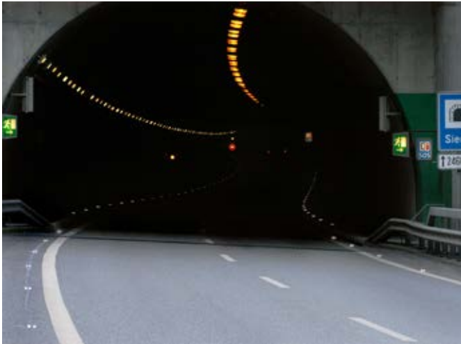
Tunnel St. Maurice, Wallis
